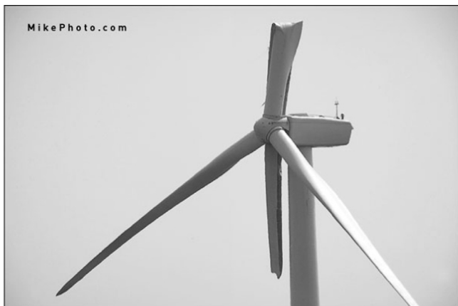
Fig. 2. Structural failure in a wind turbine blade. Photo by Mike Lascut, used with permission.
