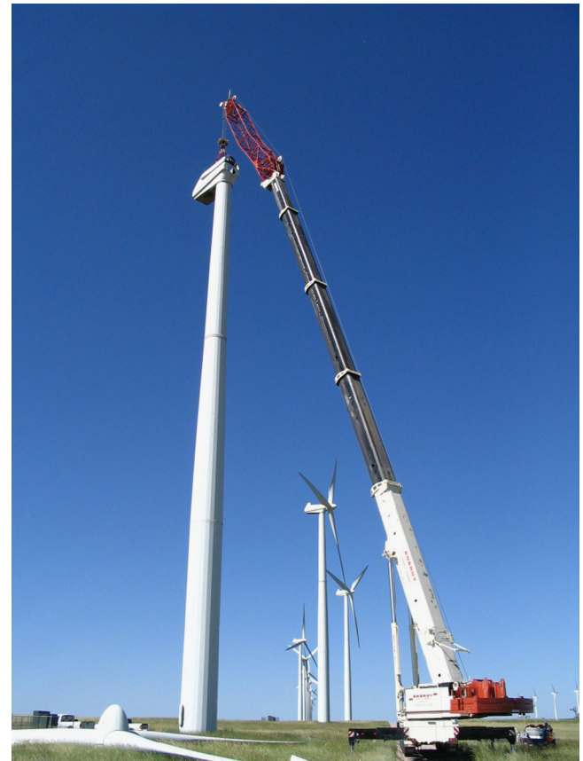
Fig. 8. Installing a gearbox. Photo by Jeroen van Dam, NREL 19257.
